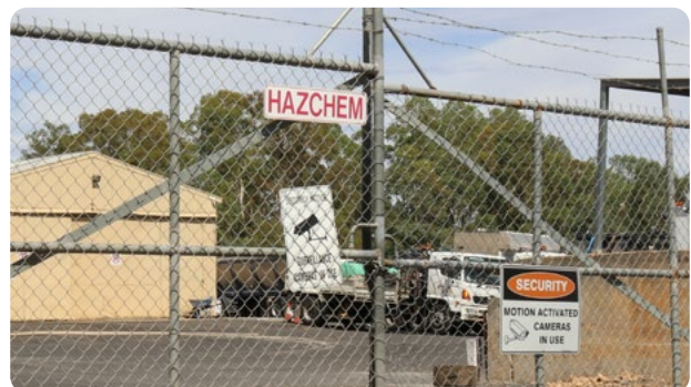
Appropriate Hazchem signage at the main entrance
