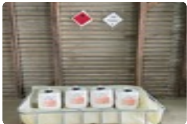
Example: Cut down shuttle used as a portable bund (for Class 3 Flammable Liquid)
